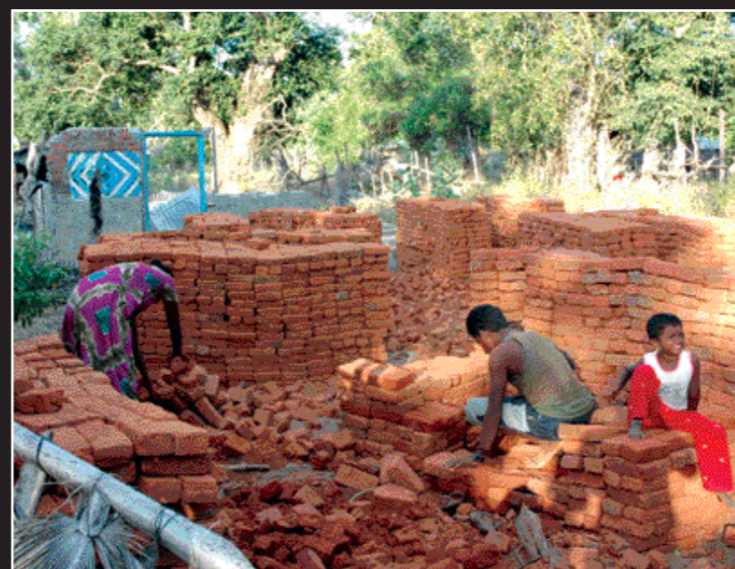
Brickmakers will now find a ready market outside Vakarai
