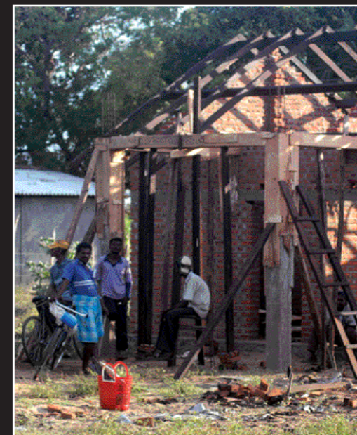
Re-construction of a house in progress
