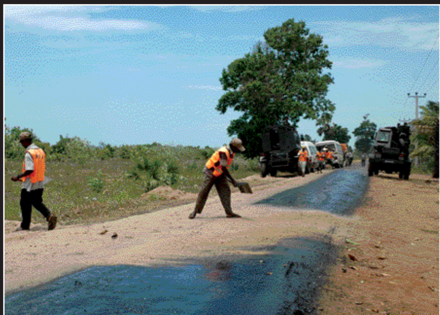
Roadways were being done up
